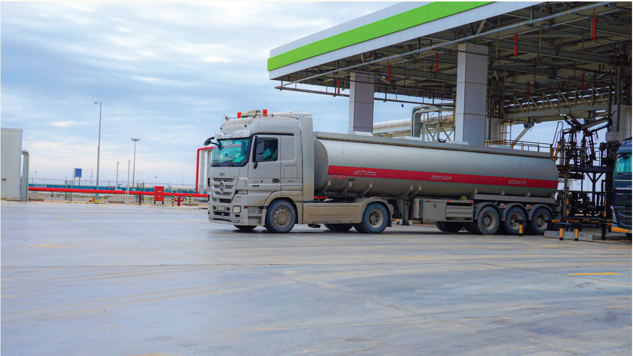
A full tanker being loaded at the Karbala Refinery. Photo credit: Karbala Refinery official website
